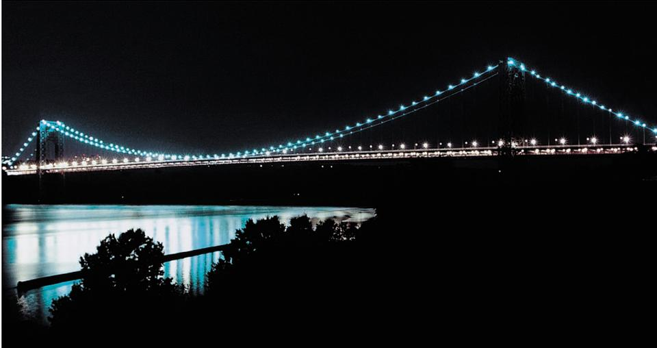
The George Washington Bridge crosses the one-mile span of the Hudson River, from the shores of Manhattan in the east to the bluffs of New Jersey's Palisades on the west side. The bridge features an upper deck with eight traffic lanes and a lower deck with six lanes. It is one of the world's busiest bridges, carrying 54 million cars annually, and the only 14-lane suspension bridge in the world.
