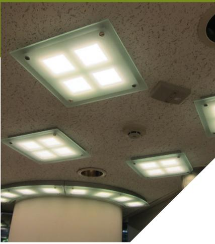
comfort for station visitors and employees. Both photocells and infrared occupancy sensors are installed to ensure ideal color temperature levels based on natural light and the number of occupants at the station. Of the 1,174 LED lighting fixtures at Jiyugaoka Station, 494 are on the platform, 238 are in the concourse, 290 are in the station office and bathroom, and 152 are in the travel center.
